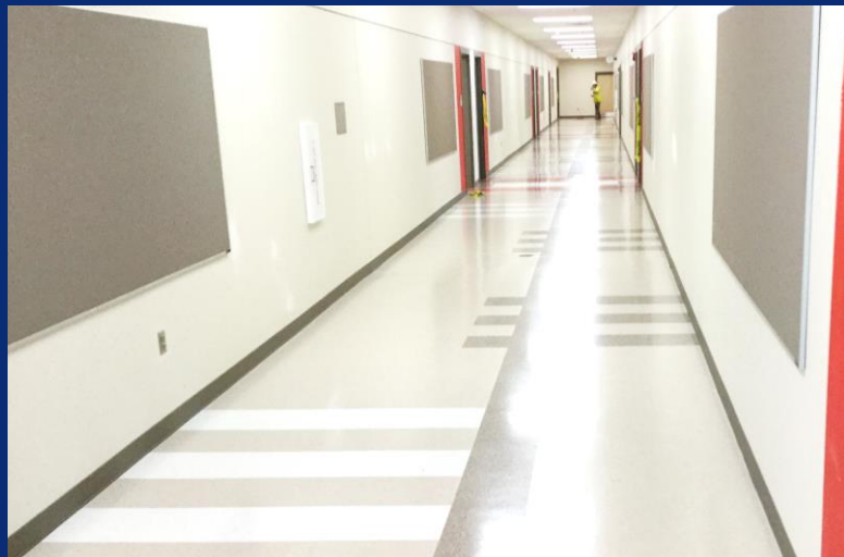
Main Level East Floor Corridor VCT Wax
