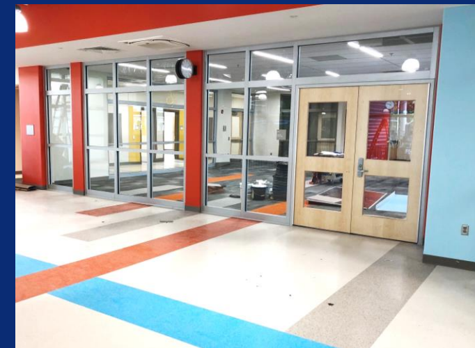
2 nd Level Lobby VCT Installation and Paint
