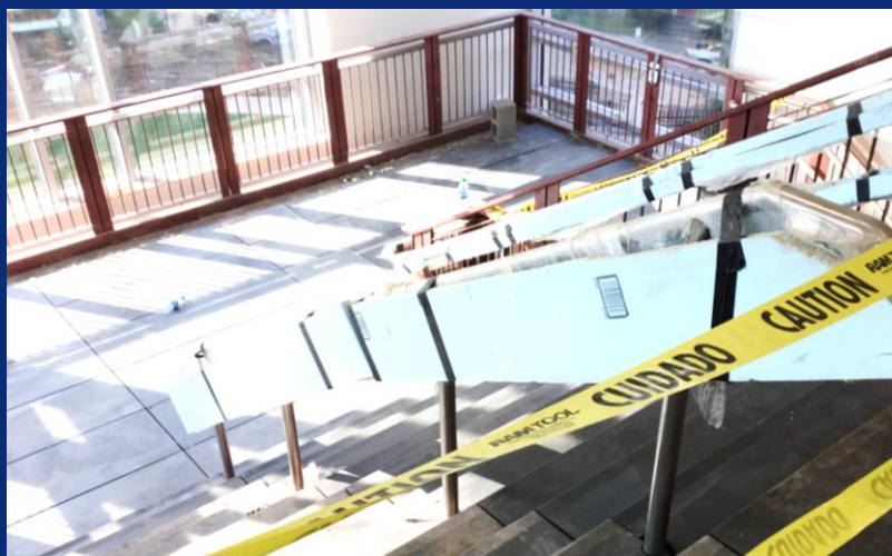
South Stair Precast Tread and Landing Install
