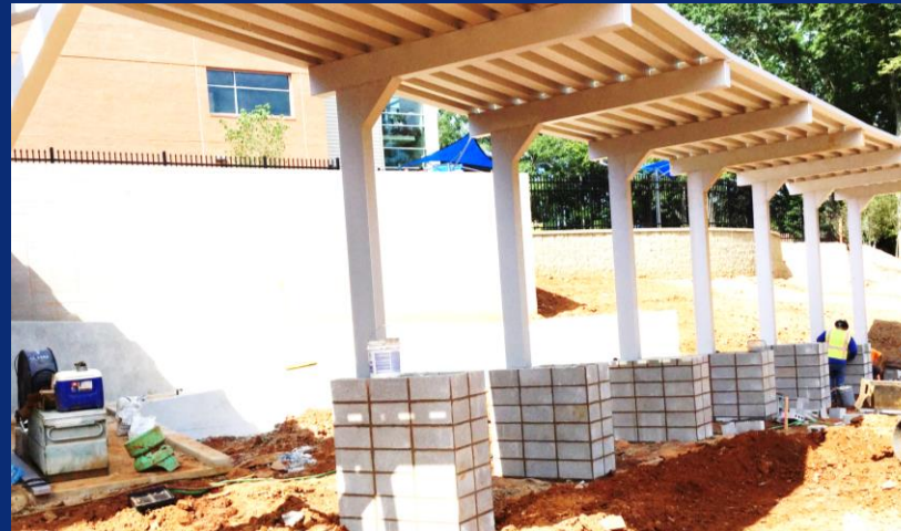
Canopy and Polished Block Column Wrap Installation
